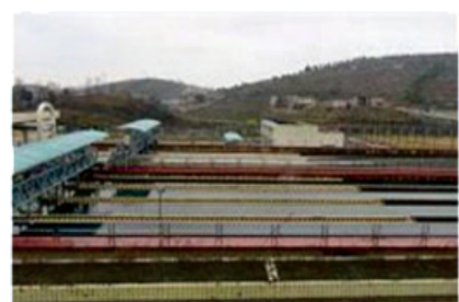
自来水厂 Tap Water Factory
