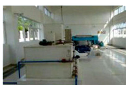
自来水厂 Tap Water Factory
