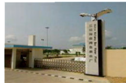
自来水厂 Tap Water Factory
